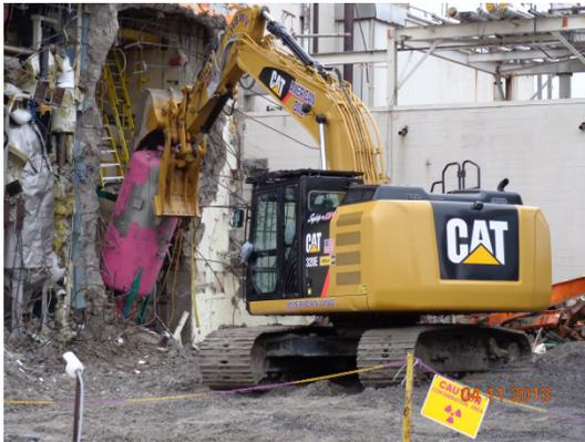
High-visibility paint will be used to identify equipment that requires special handling during demolition. This practice safeguards against unintended radiological releases and maximizes operator distance from radioactive materials. These measures were successfully demonstrated during demolition of the contaminated 01-14 Building at the WVDP in 2013.
