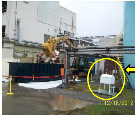
Waste debris packaging at the point of generation is one method used to control contamination. Air monitors located in the cab of the demolition equipment and in stand-alone ground units like the one outlined in the foreground above will monitor the demolition area for any unintended airborne disturbance.
