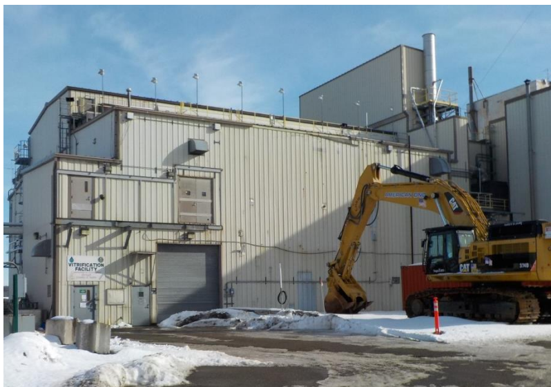
The Vitrification Facility was used at the WVDP to vitrify radioactive HLW into glass.
