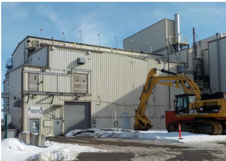
**The WVDP Vitrification Facility was used to vitrify radioactive HLW into glass.**
