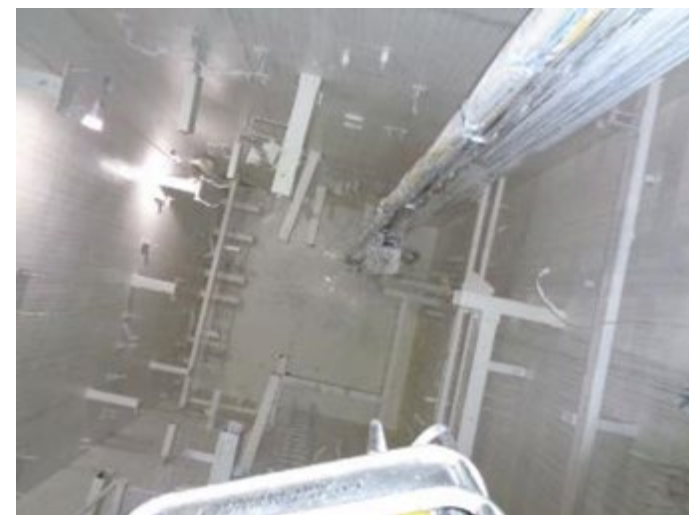
Extraction Cell-1 After Deactivation
