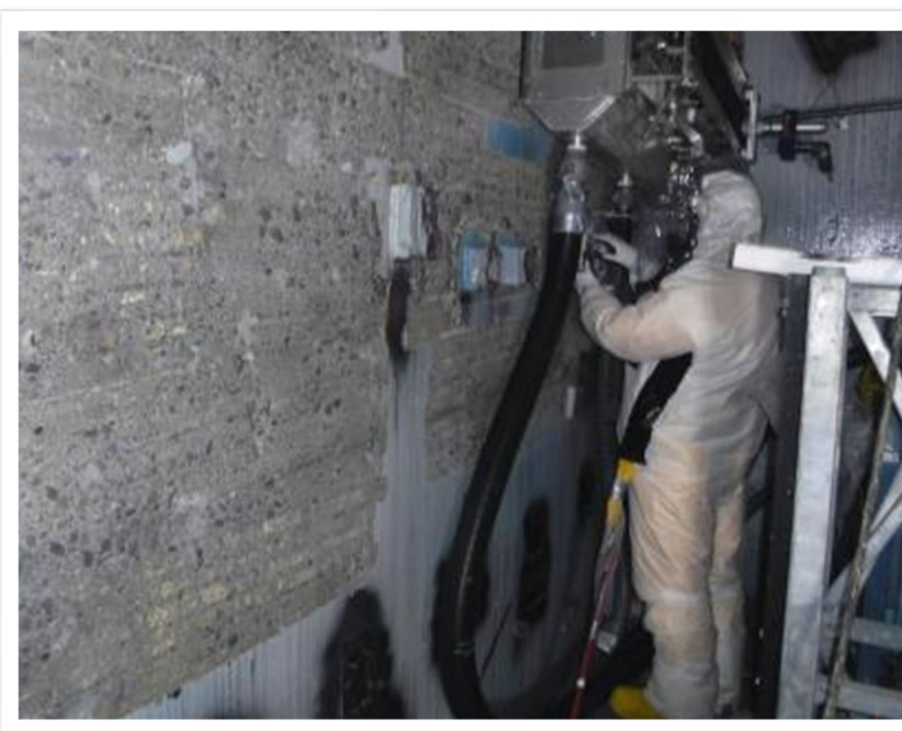
Radiological surveys are taken on the south wall of the PPC-S, after decontamination
