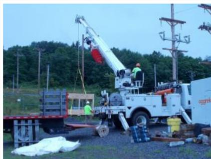
Workers install a new electrical recloser on the site's new switchgear station. The recloser will act like a circuit breaker if the system experiences any type of electrical interruption.
