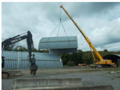
A large crane is used to relocate sections of the CPC-WSA to an area where they can be safely demolished.
