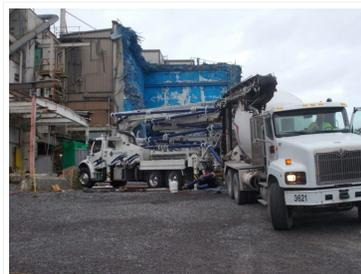
A pumper truck is used to place grout into the general purpose cell of the main plant process building at the West Valley Demonstration Project. The grout will provide structural stability to allow heavy demolition equipment to drive over the below grade rooms, while the main plant process building is being demolished.
