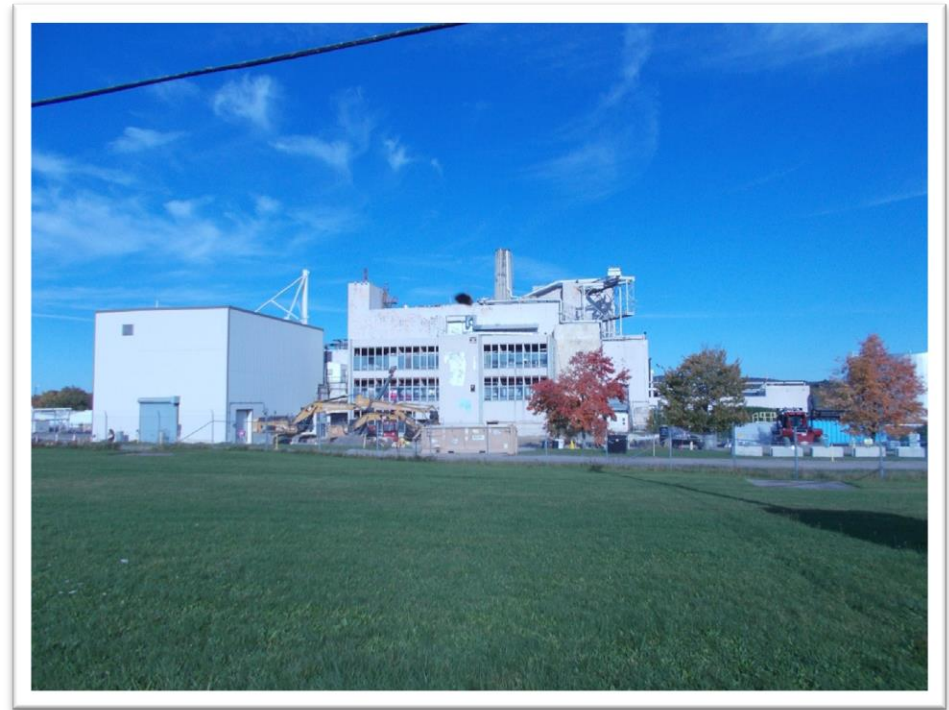
Main Plant Process Building
