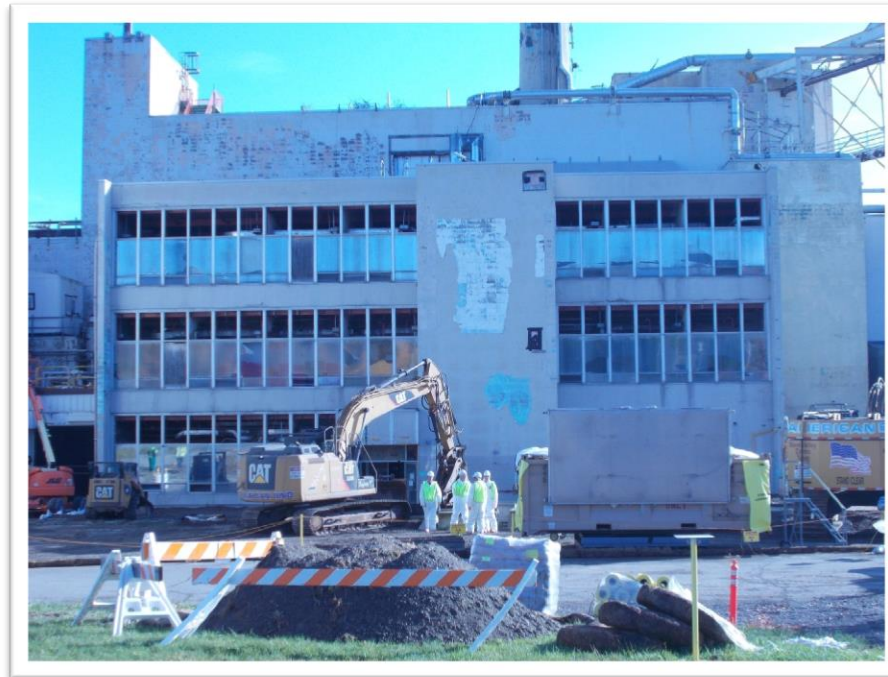
Main Plant Process Building (pre-demolition of Office Building)
