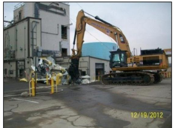
**Figure 2: Removal of the uncontaminated outer portions of the building.**
