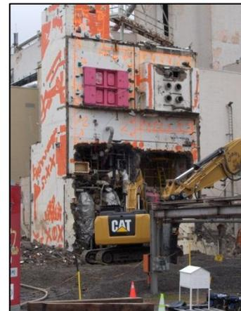
**Figure 4: Demolishing the contaminated portion of the 01-14 Building.**
