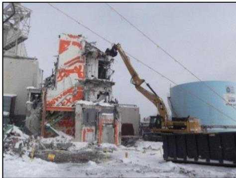
**Figure 3: Removal of the uncontaminated roof and concrete walls.**
