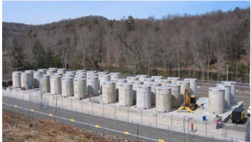
*The West Valley HLW Storage Pad is an exterior reinforced concrete structure designed to bear the weight of more than 50 concrete storage casks containing vitrified (glass) radioactive high-level waste. The storage area is located on the WVDP site and will appear similar to the one pictured above.*
